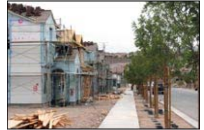
Construction continues at Inspirada in Henderson.
