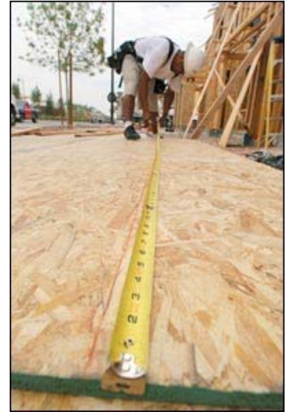
Carpenter Javier Espinoza frames a home under construction at the master-planned community Inspirada in Henderson.
