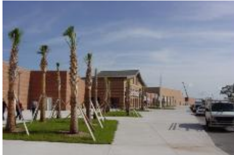
Growth in Manatee County may require building more schools like this one, Braden River High School.
