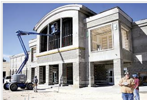
Foreman Chris Millican (foreground) of Division 9 Construction Inc., of Rome, Ga., oversees construction of the 45,000-square-foot Publix Supermarket located in the new Lake City Commons shopping center. JASON MATTHEW WALKER/Lake City Reporter
